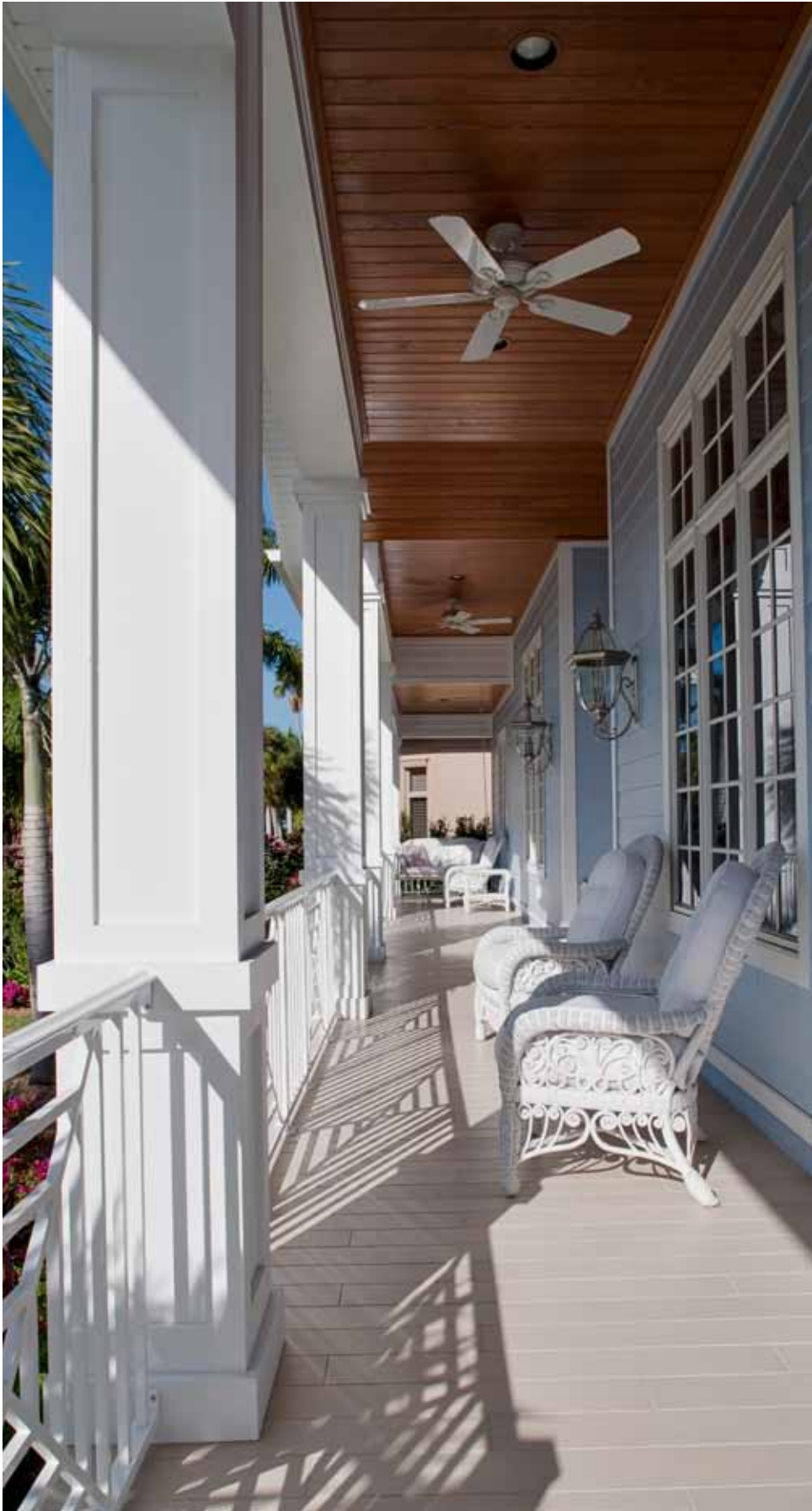
Naples - Old Naples Custom Home - Front Porch
